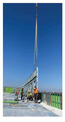
To build the towers, 202 tractor trailers delivered 3,134 panels manufactured locally from coil stock by Klover Contracting. Just-in-time delivery was used and panels were picked directly from the trucks by tower cranes.
