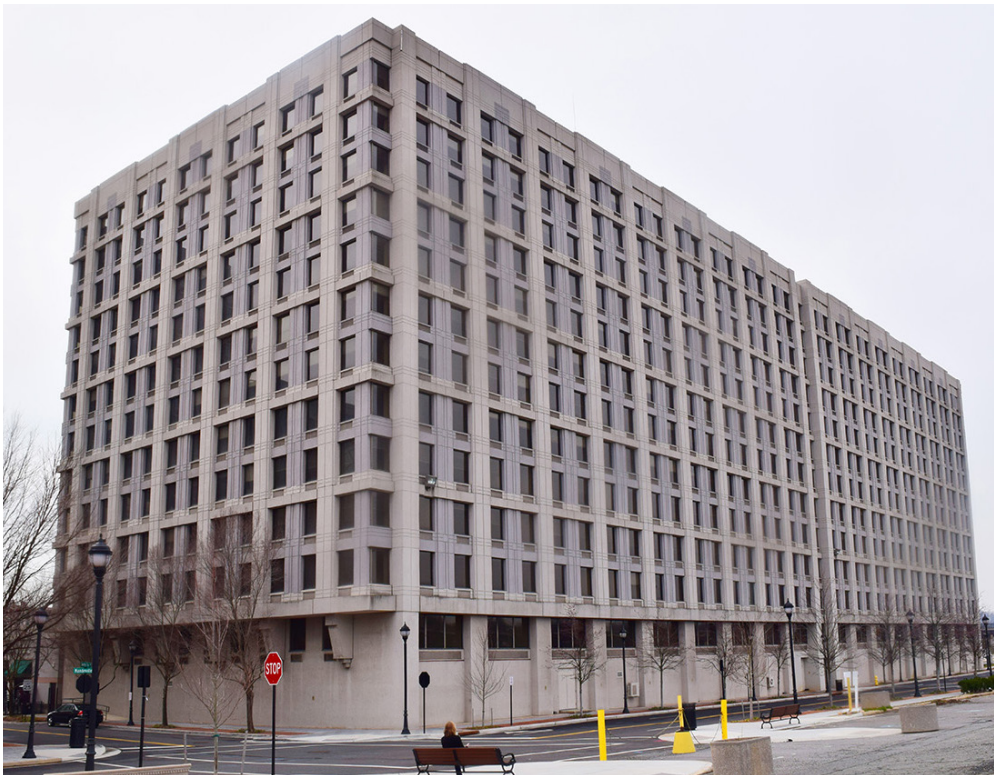
Photo courtesy Cooper Carry
